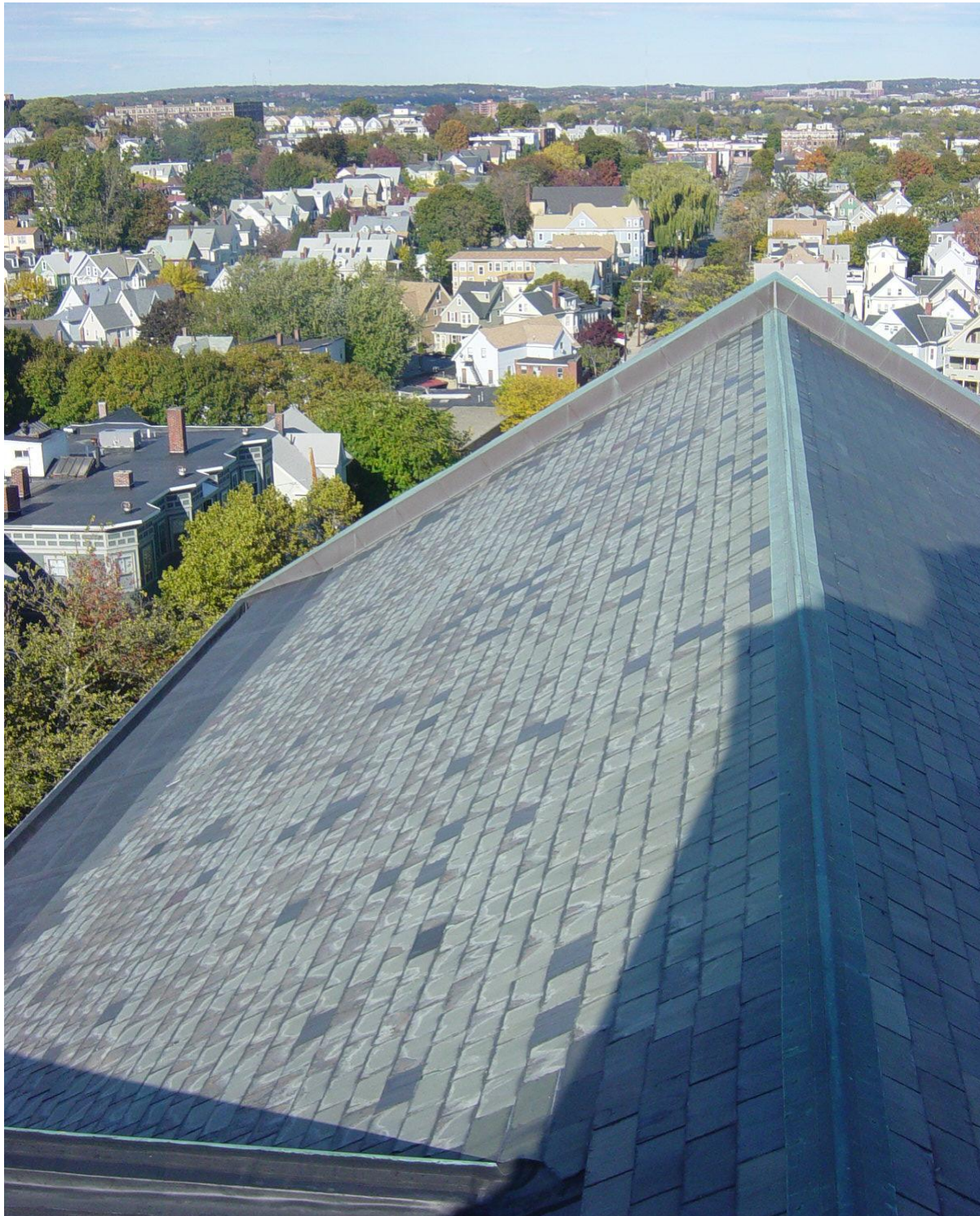
Photo 15 - Slate roofs are in good condition. A few cracked and missing slates were seen. Built-in EPDM lined gutters appear in good condition. The copper ridge appears to be in good condition.
