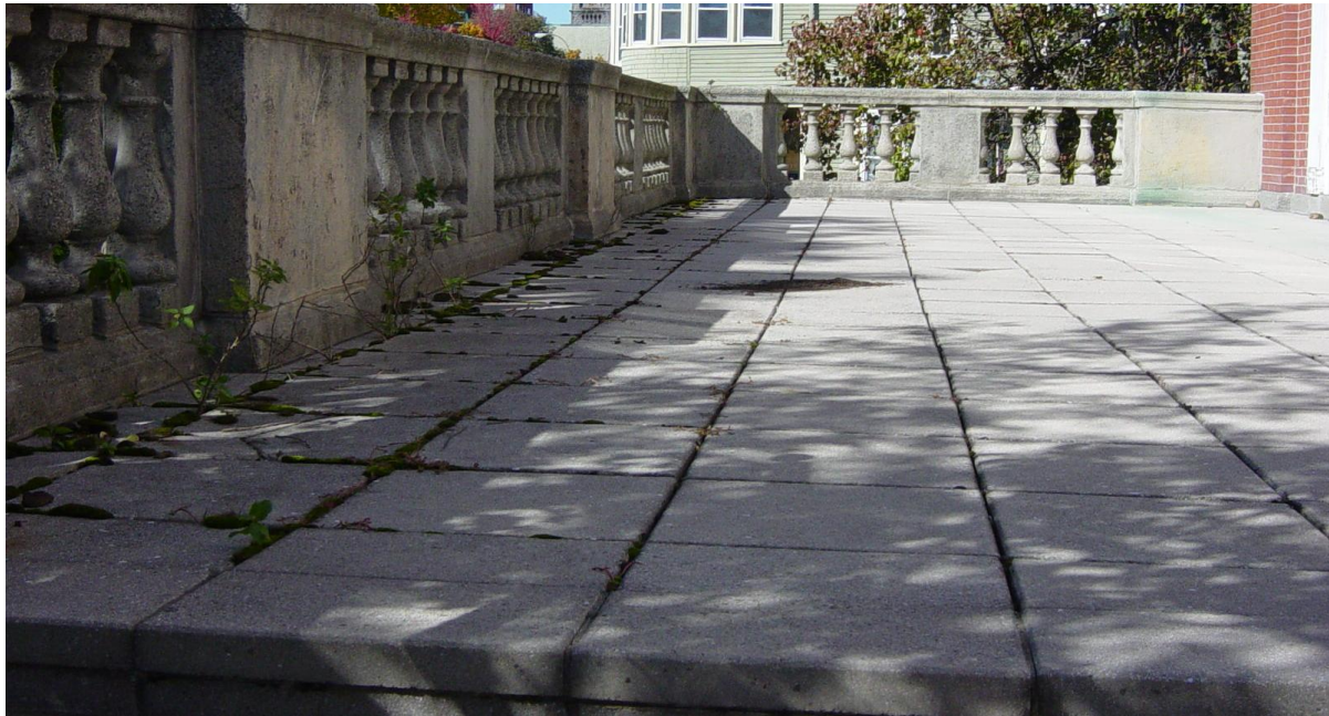
Photo 9 - Terrace waterproofing is failing, causing water and tar leakage at offices below. Moss and plant growth is seen and should be removed for proper function of terrace drains. Some deterioration of the cast stone guardrail was seen.
