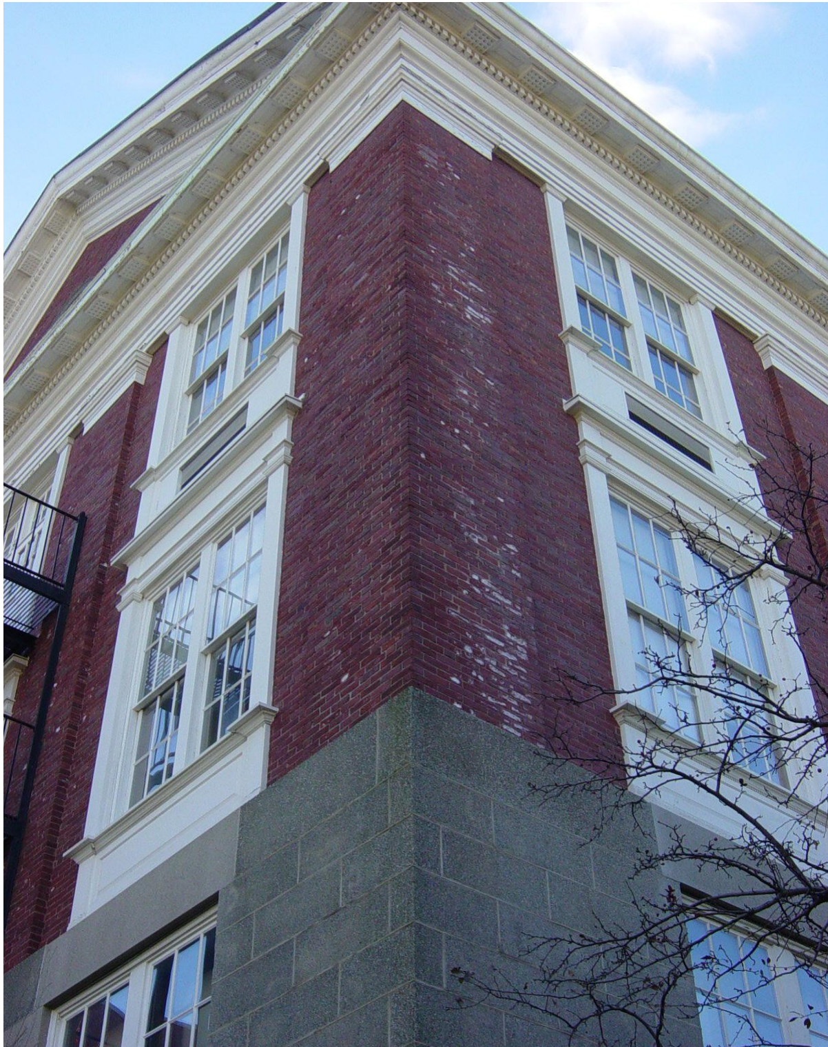
Photo 11 - Brick walls, granite base and building mortar are in good condition. No settling or cracking of masonry was seen. Due to weather, the northwest corner of building showed the most deterioration to the
