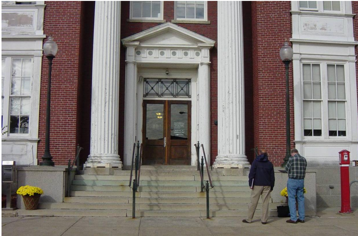
Photo 1 - Sealant is badly deteriorated at granite steps of Main Entry. Handrails are scratched and rusting. Painted columns, window and door surrounds are in poor condition.
