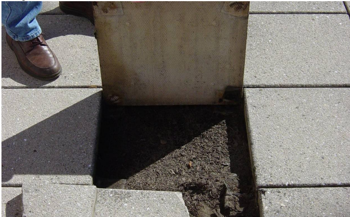
Photo 10 - Terrace pavers need to be removed to clean out organic debris, which is clogging the drains. Some pavers are cracked and need to be replaced. Drain pipes need to be insulated to prevent sweating.
