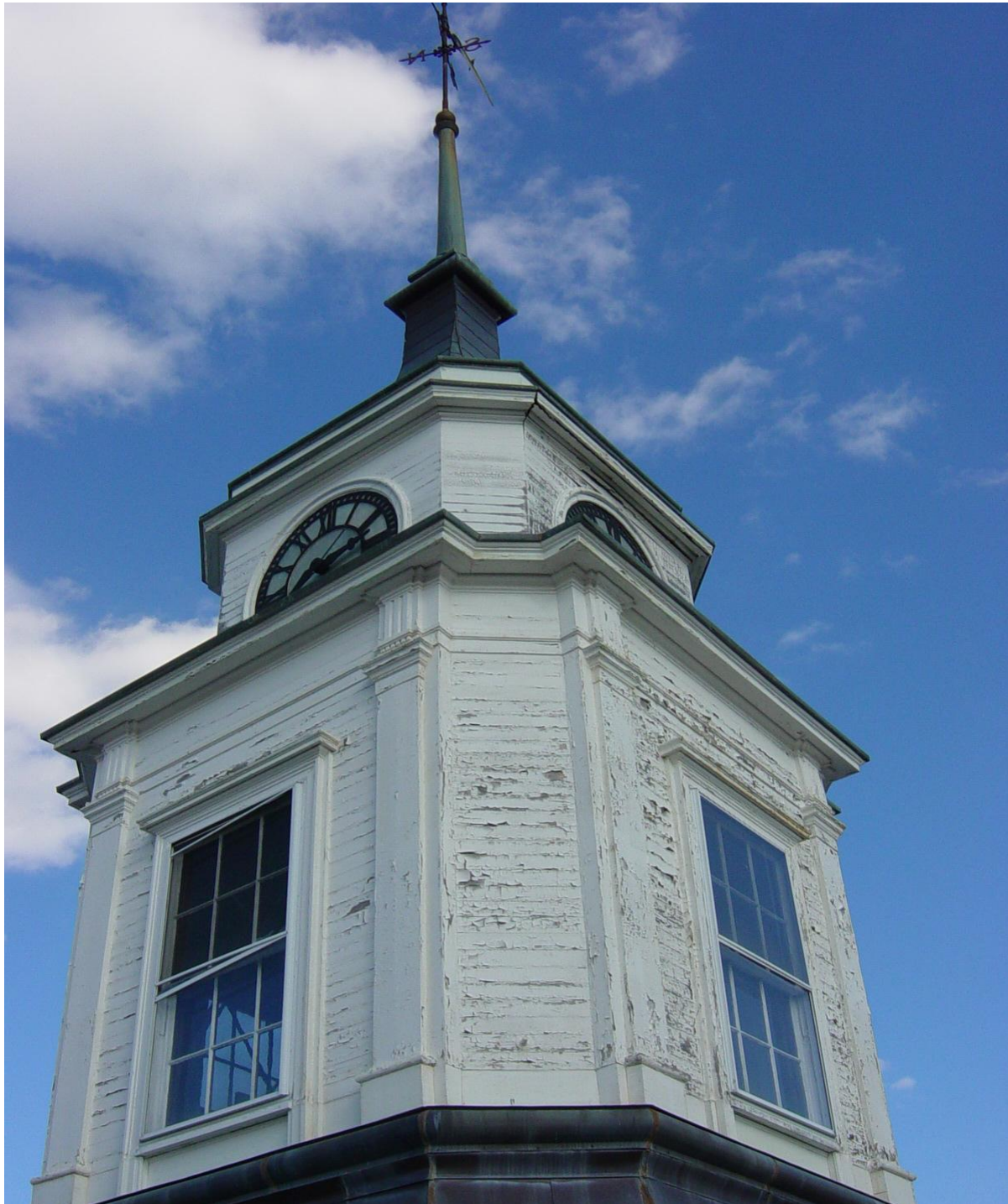
Photo 23 - The clock tower paint is peeling badly. Some wood trim is loose and in need of repair. Windows are in very poor condition. They have not been fitted with insulated glazing as was done elsewhere. Non-historic storm windows have been shattered due to high winds. The copper roofs appear to be in good condition, and no water was seen leaking from the steeple in moderate to heavy rains.
