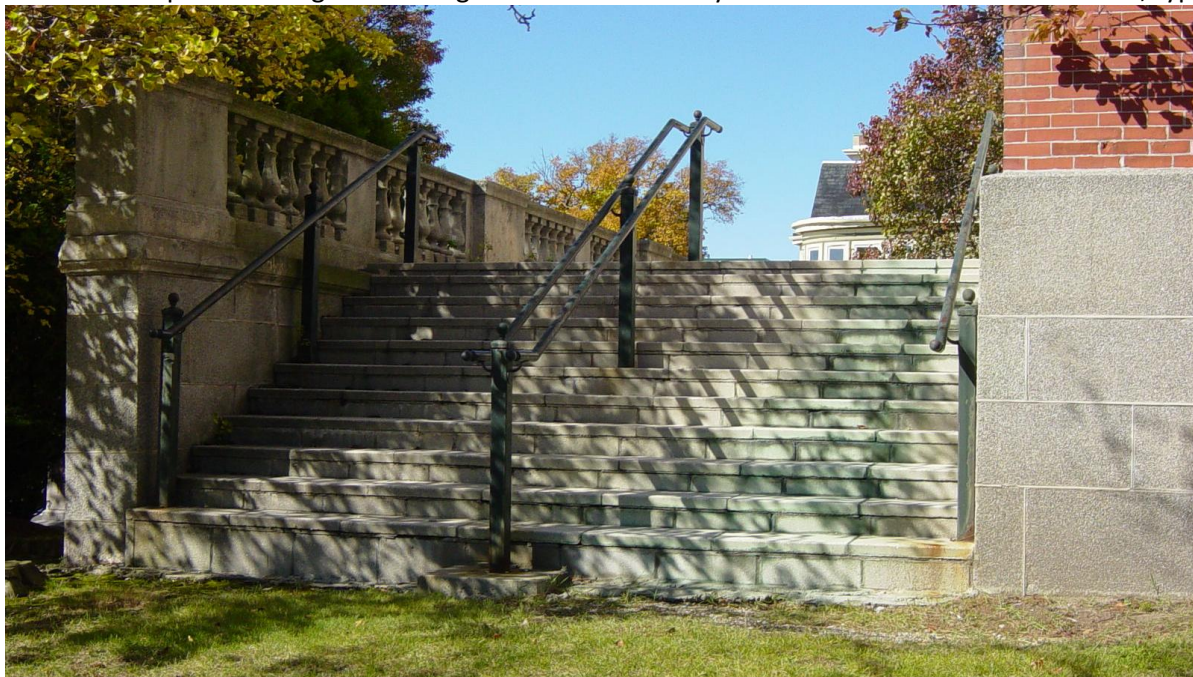
Photo 8 - Riser at bottom step is too high. Build up grade below steps to make bottom riser equal to others.
