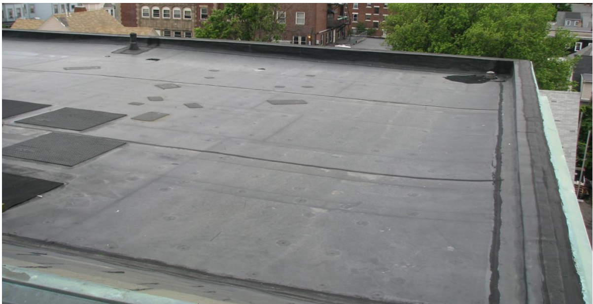
Photo 17 - The flat EPDM roofs are approximately 19 years old and in fair to good condition. Some roof drains are damaged and in need of repair.
