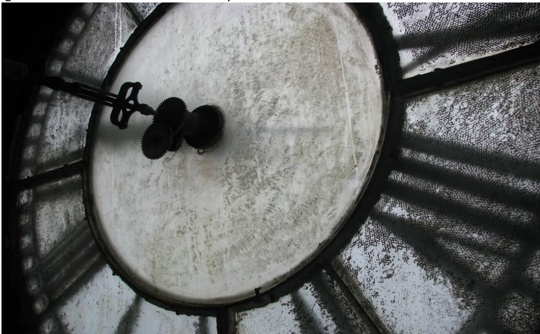
Photo 2 - The clock is not functioning. Deteriorating glazing compound around dial may leak water.
