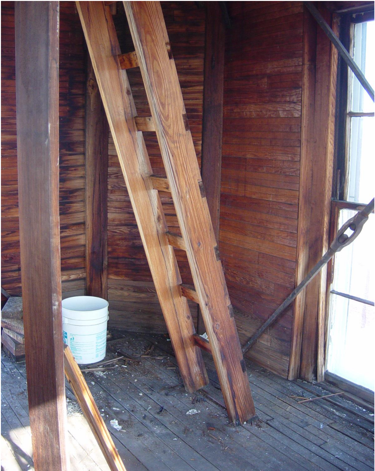
Photo 25 - Ladder to clock room is unsafe, some rungs are loose and it does not meet OSHA standards. Walls and floors are water damaged. Windows are rotted and leak. Floors are littered with debris.
