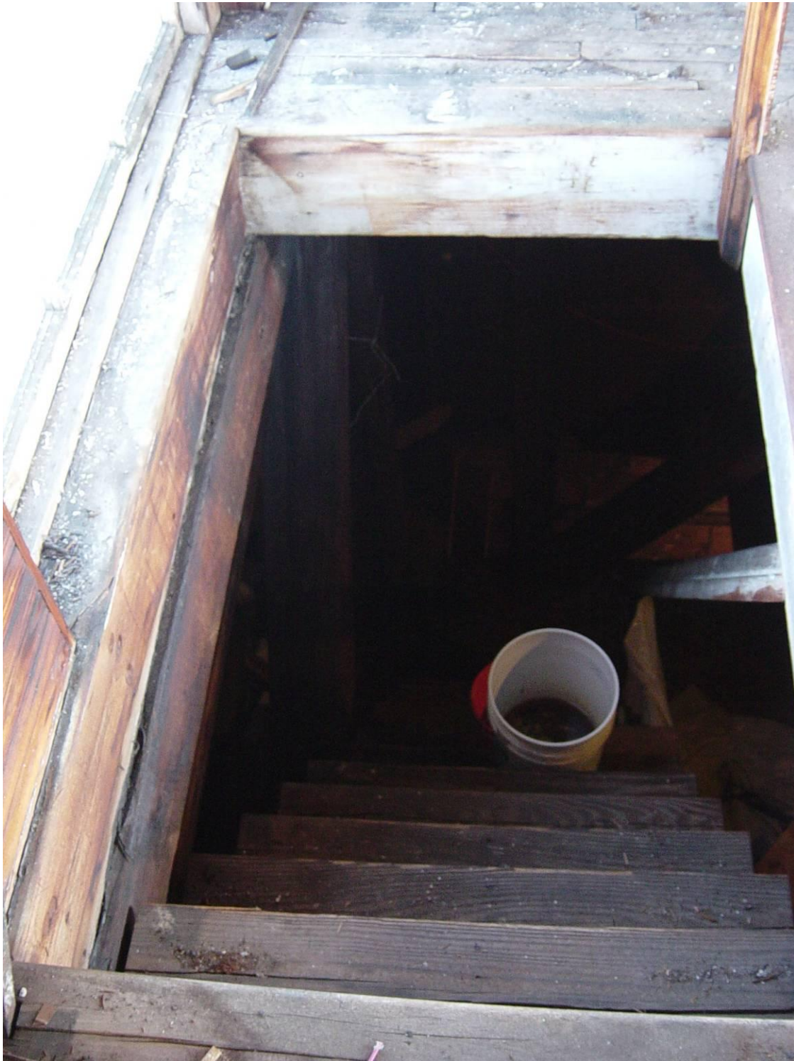
Photo 24- The stairs ascending the clock tower are very steep, with loose, cracked treads and inadequate railings. Buckets are propped to catch leaks.
