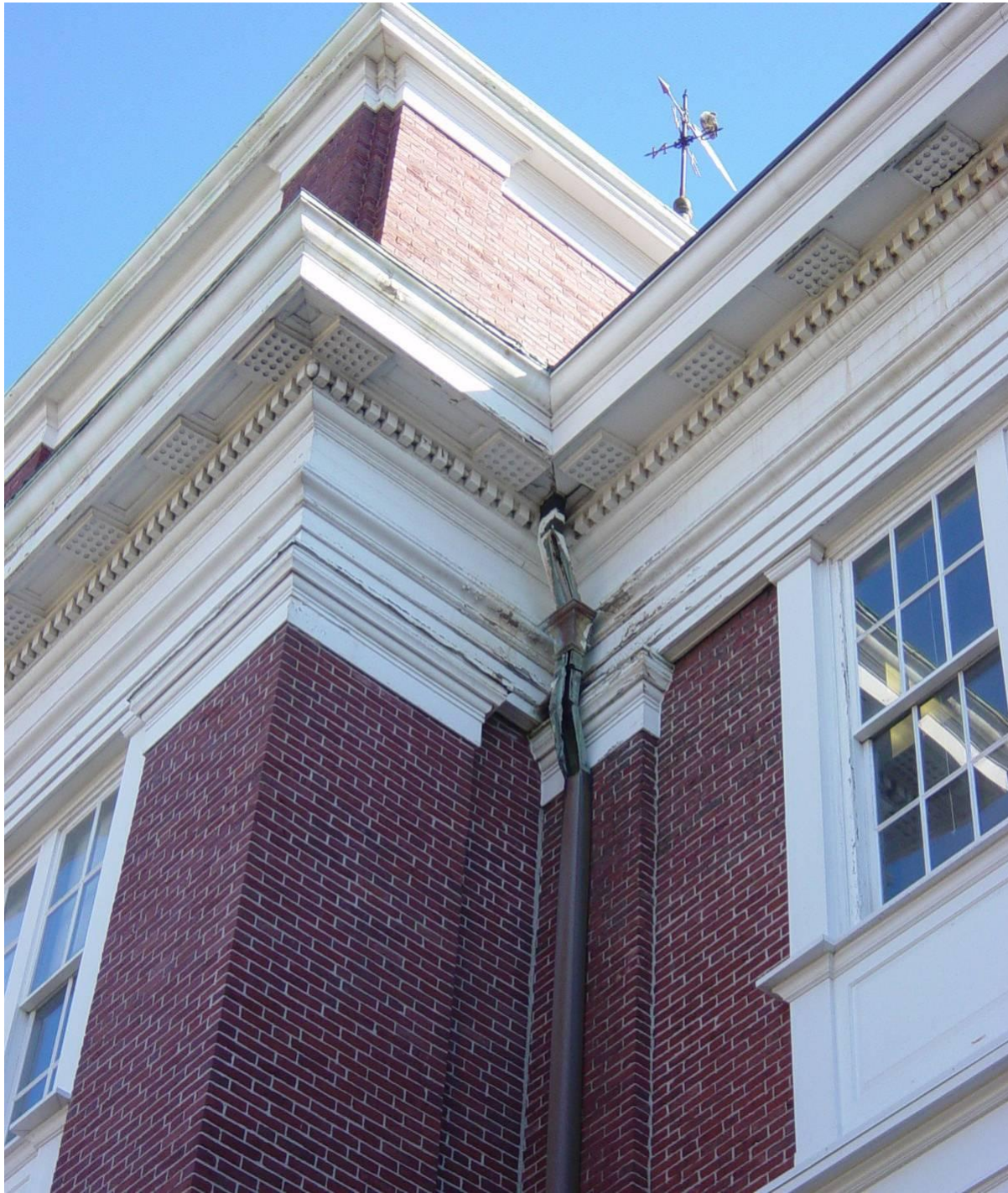
Photo 13 - Paint at wood cornices and other wood trim is peeling, in some cases badly. Some copper downspouts have split, causing large amounts of water to spill down the face of the building. Below this downspout, which is adjacent to the Accounting Office, water has damaged the interior wall surface.
