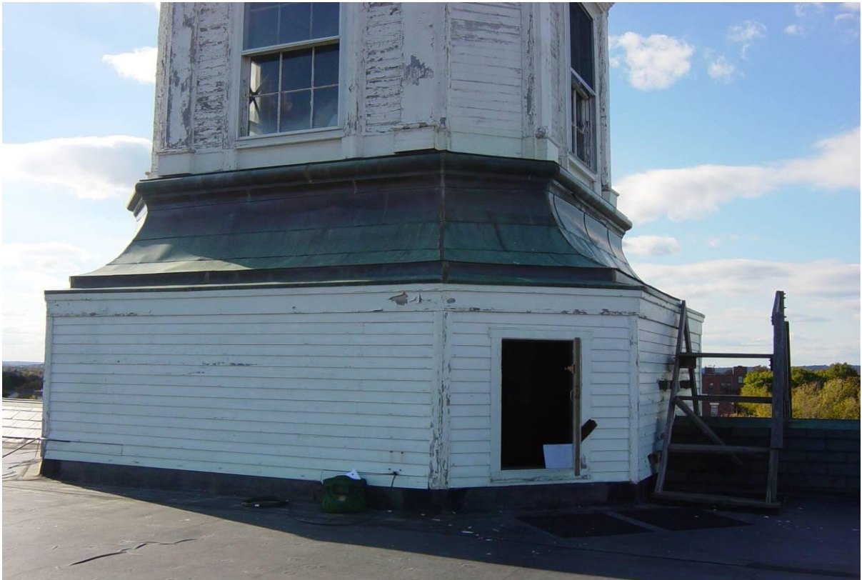
Photo 22 - The clock tower is clad in painted clapboard, wood trim and copper roofing. It has three floor levels, the lowest of which exits onto the flat roof. The crossover stairs on the right are used for accessing the west roof and mechanical equipment. It is missing treads, poorly built and hazardous. Replacement is recommended.
