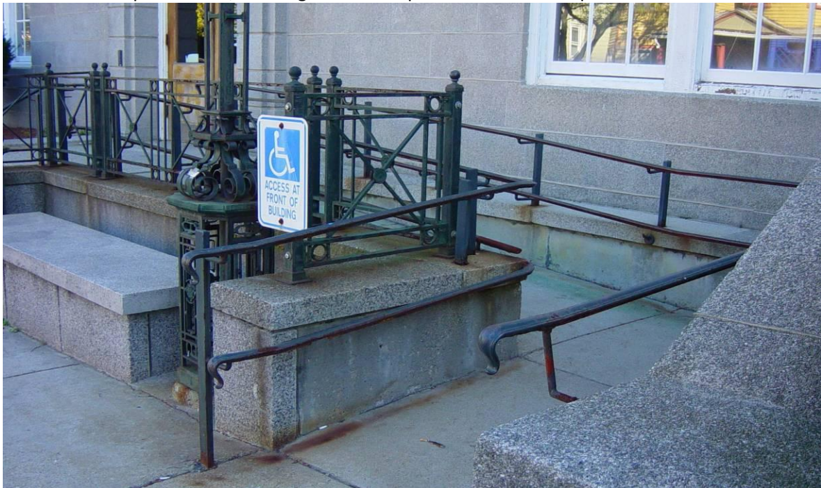
Photo 6 - Ramp to basement does not meet Accessibility Code (MAAB). Ramp is too narrow and railing profiles do not conform. Ramp posts are loose.
