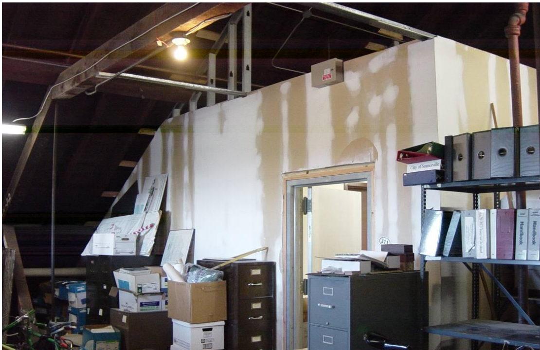
Photo 21 - Attic is currently crammed with old files and drawings. Tension rods and braces obstruct space.
