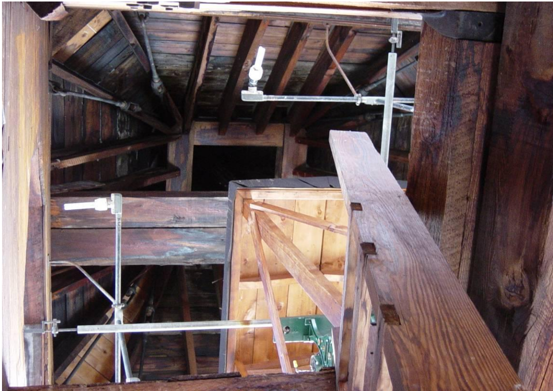
Photo 26 - Timber frame and tension rods appear to be in good condition. Some rot is seen at the roof planks. It is not clear if this is recent, and may be due to condensation rather than leakage. No roof leakage was observed in moderate to heavy rain and winds.
