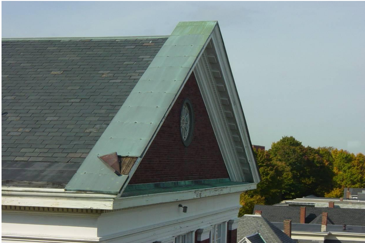
Photo 16 - Several areas of the copper coping are damaged and in need of repair.
