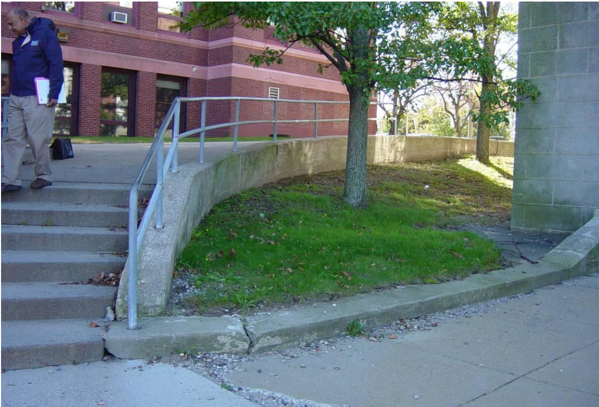
Photo 3 - Concrete retaining wall is beginning to lean, but not showing signs of imminent failure.
