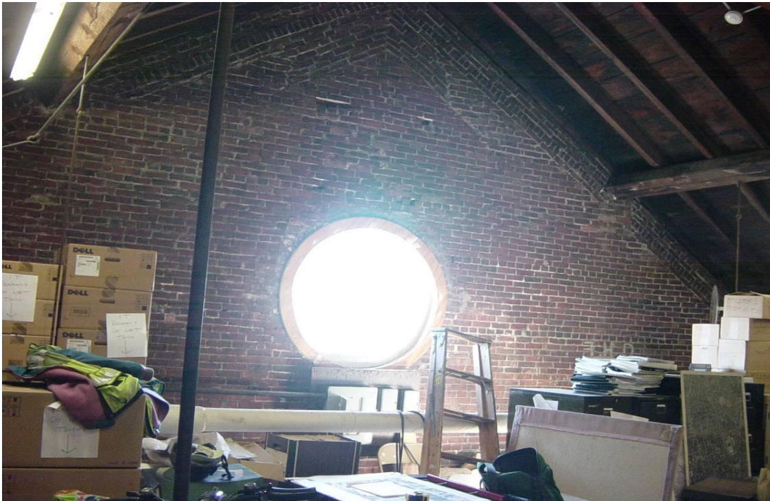
Photo 20 - Existing south attic has exposed brick wall, window and roof timbers. Steam pipes obstruct space.
