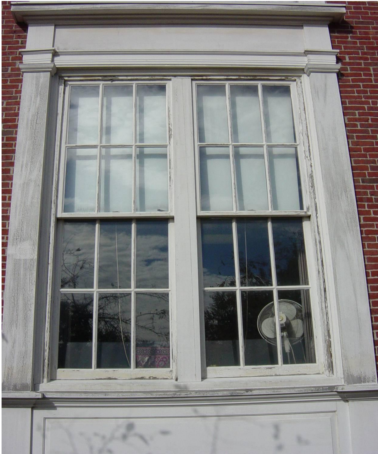
Photo 14 - Windows are single hung, wood sashes and frames retrofitted with insulated glazing and weather stripping. The condition of the windows is good, but the sashes have excessive play, some weather stripping is missing, the glazing compound is cracking, and painting is needed.
